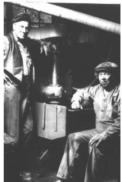
The first vertical pump, manufactured 1933.
