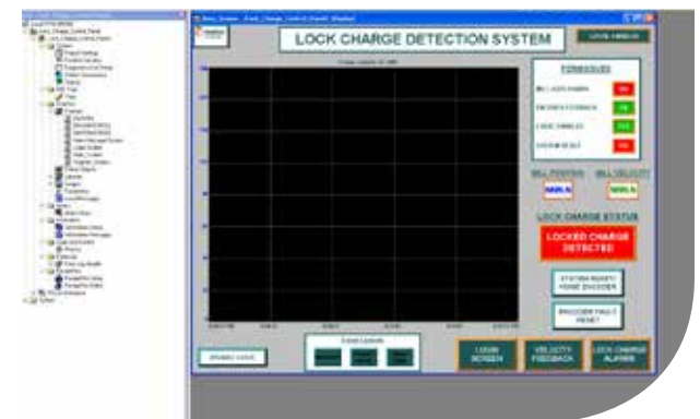
Locked charge detection system screen
